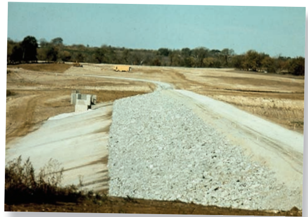
Building a dam is no small job. Gravel road atop newly constructed dam.
