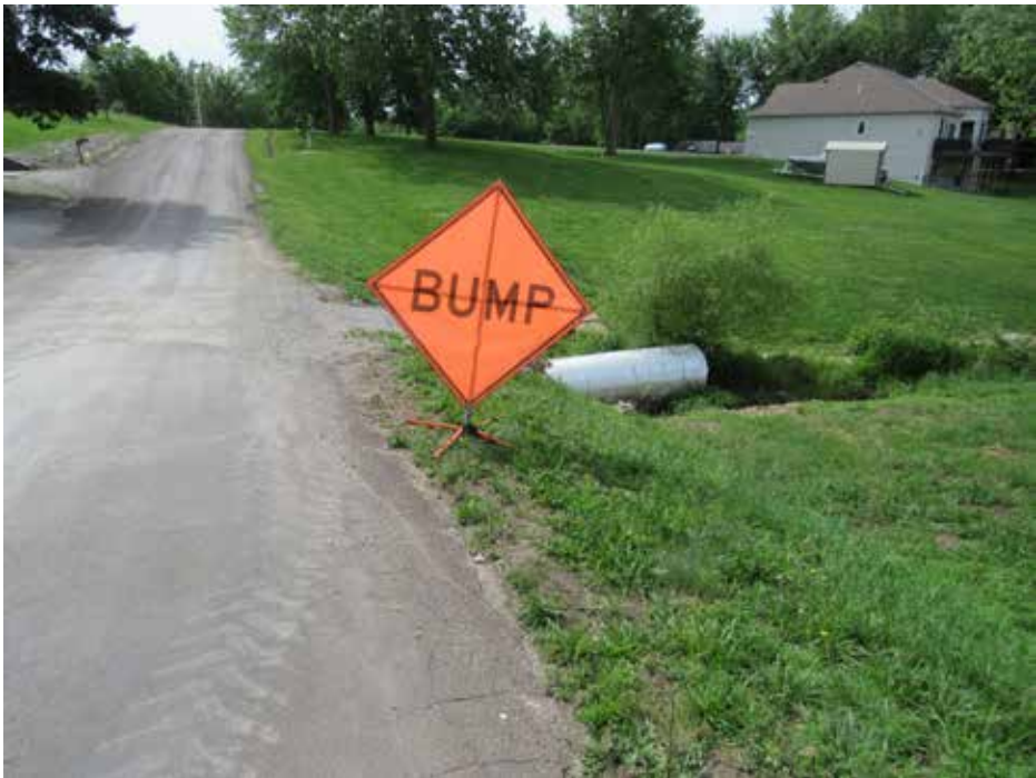
A few bumps in the road mean that the Association is doing tube re-placements as part of the scheduled maintenance program.
