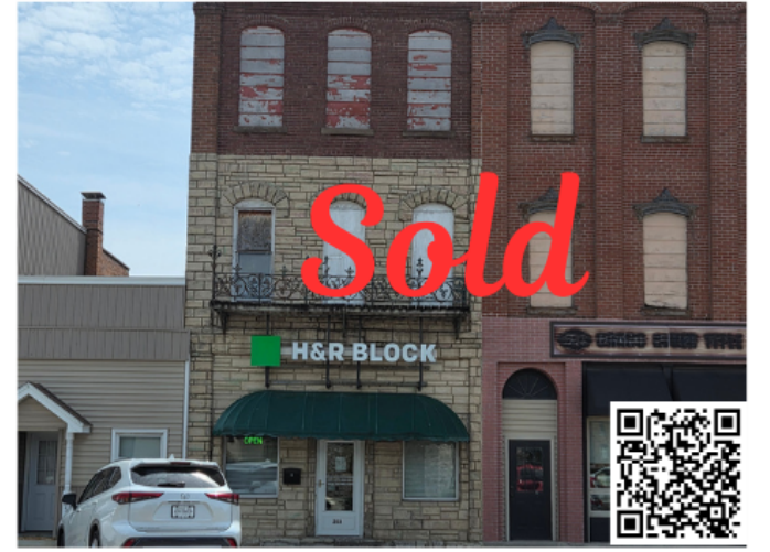
Sold 203 N. Main Gallatin, MO. 64640 $120,000. Commercial Building. 1 st floor leased $800 month
